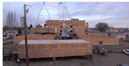
Fig.1. Modular building construction using mobile crane
