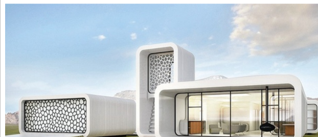
First 3D printed model in Dubai The building uses Chinese company WinSun's tilt-up technology, where the floor, walls and ceiling are all 3D printed. It's the world's first 3D printed building. Ideally, the printer would be located at the job site in Dubai, but in this case it was built in WinSun's factory in China. The modules were cut in half so that they could be shipped more easily and reassembled on site.
