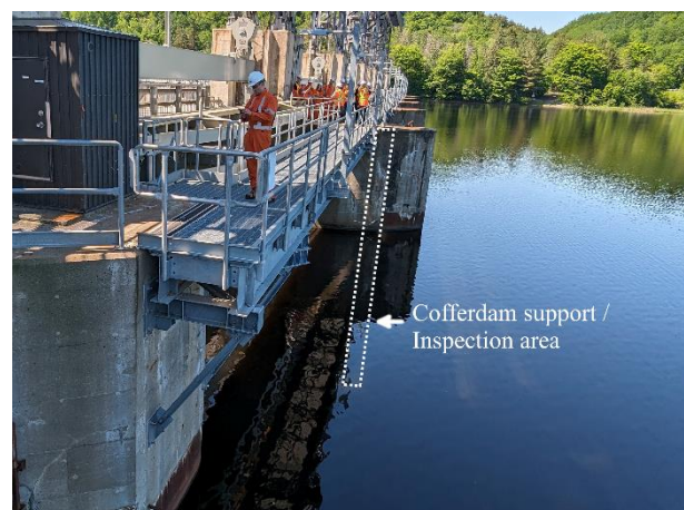
Figure 1. La Gabelle dam, upstream view of the concrete piers and inspection areas.
