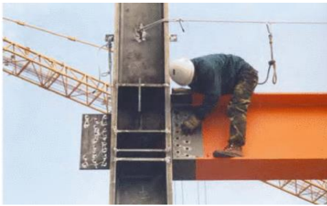
Figure 1 Safety risks of a human working at height during steel building construction [5]
