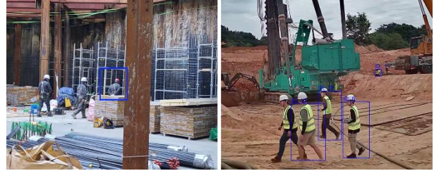
Figure 10. Challenging Cases in Real-world Construction Sites
