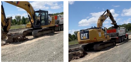
Figure 2. Left Image: Excavator idle, and right image: Excavator and truck working in tandem
