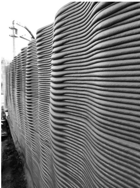
Figure 5. Perspective detail view of 3DPC Walls.
