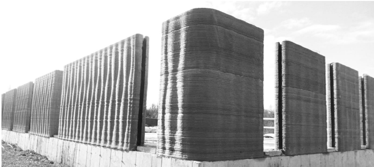
Figure 4. Perspective view of 3DPC Walls.
