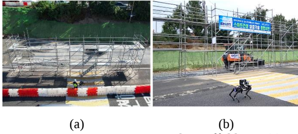
Figure 3. Data acquisition at the scaffold site; (a) scaffold site where point cloud data were acquired, and (b) quadruped robot used for data acquisition.
