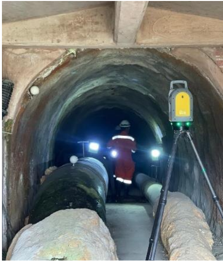
Figure 2. Data acquisition process inside the tunnel.
