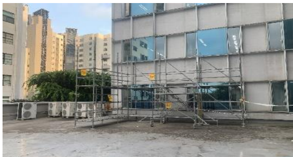
Figure 4. Scaffold installation at ConTIL Laboratory
