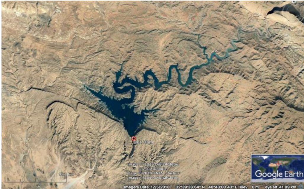
Figure 3. Dez dam study area
