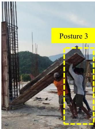
Figure 5. Panel erection
