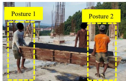
Figure 4. Panel lifting
