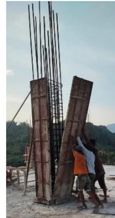
Figure 3. Workers erecting formwork panels around the rebar
