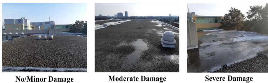
Fig. 3: Examples of the Collected Images Representing the Three Different Damage Categories
