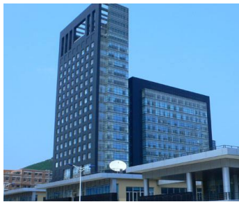
Figure 4 Creative Plaza building
