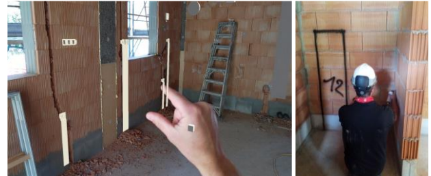
Figure 1. Marking works with the AR HMD (Trimble XR10 - Microsoft HoloLens II)
