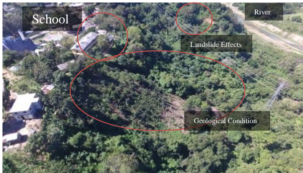
Figure 1. Community site near landslide effects
