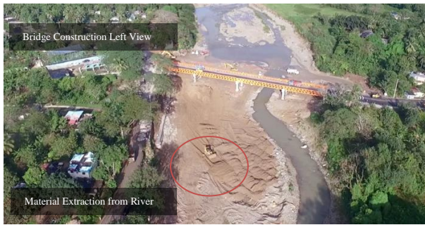
Figure 6. Construction site of the Bridge
