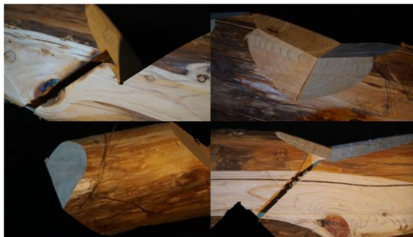
Figure 15 Enlarged view of diagonally placed components of the staircase.
