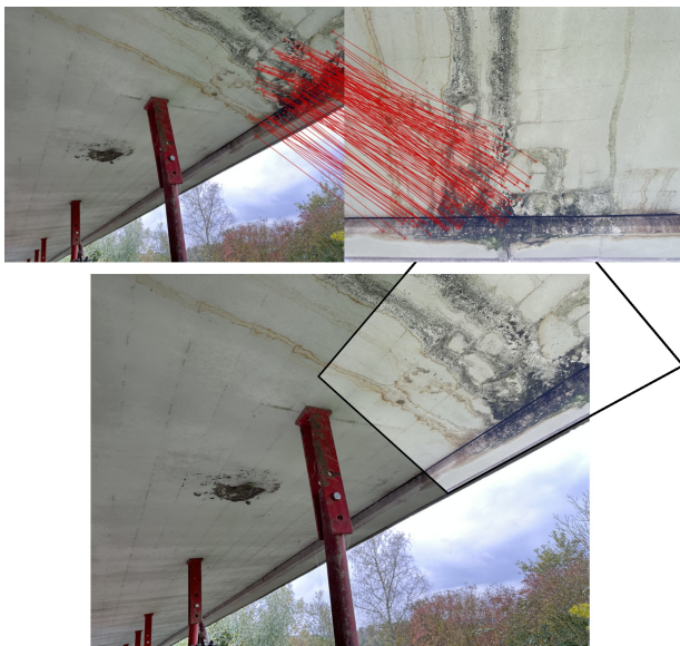
Figure 7. Example of a positive match of two images of the same defect, one with context, one with detail.
