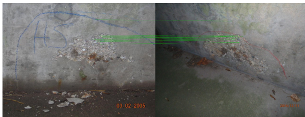
Figure 9. Example of a match between two images of the same defect, taken in 2005 and 2014 respectively.
