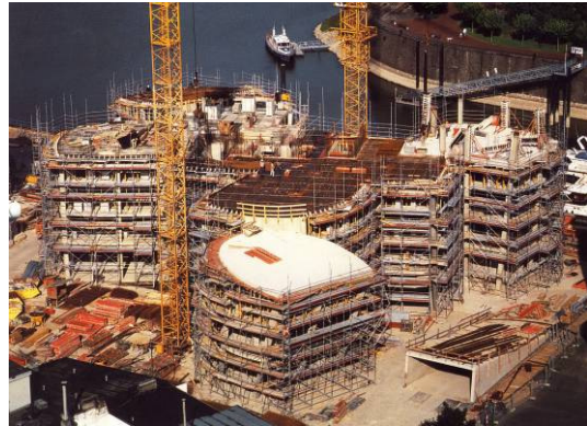
Figure 18. Structural works House C „Bodenseekiesel“ [3]
