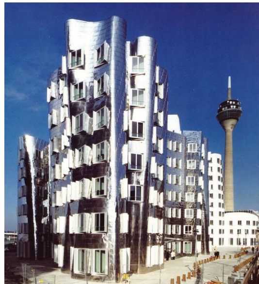
Figure 11. House B stainless steel facade [3]
