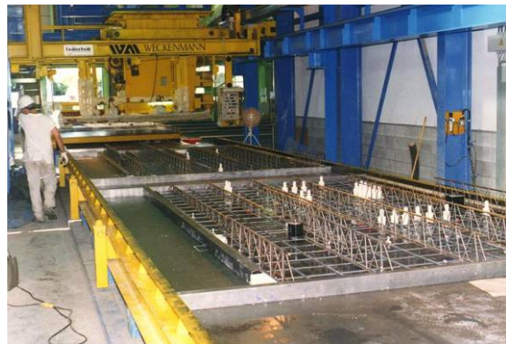
Figure 6. Pallet in concreting station [1]
