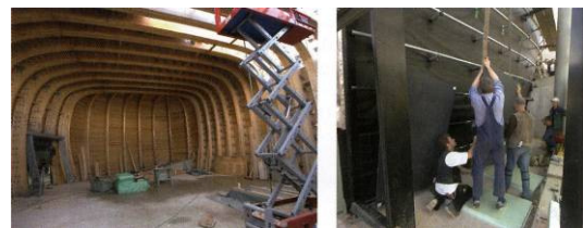
Figure 25. Inside of the wood structure and construction of the facade-elements [5]
