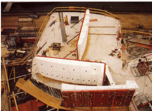
Figure 17. The reinforcement is placed in front of a formwork element, prepared wall formwork [3]
