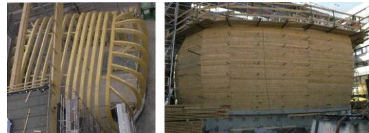
Figure 24. Assembly of the wood structure [5]
