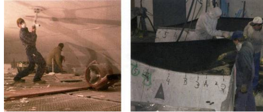
Figure 23. Modelling of the pebble-form in the igloo; production of the fiberglass-concrete elements [5]
