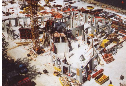
Figure 15. First floor: just-in-time assembly of the elements [3]
