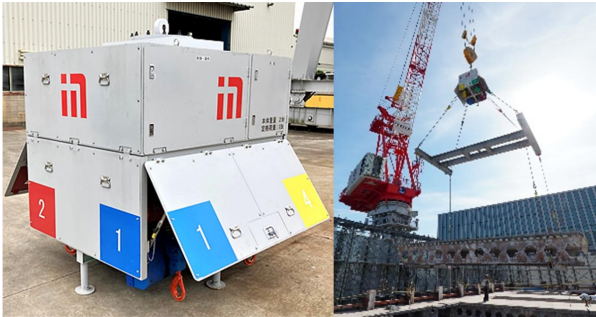
Fig.18. Four-Point Automatic Lifting Device and Slab Hoisting Condition
