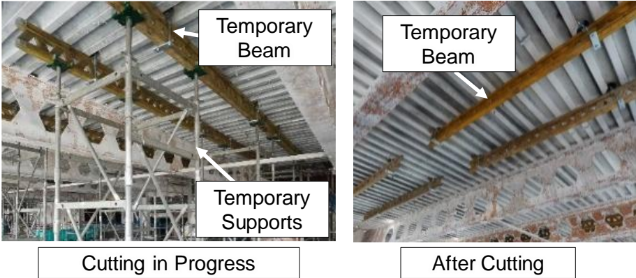
Fig.16. Lower slab before and after cutting
