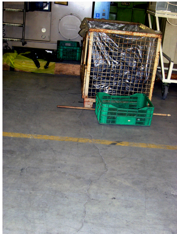
Figure 5. The damage of the industrial floor in the building
