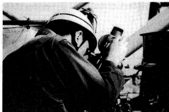
Photo 2 Plumbing and positioning of steel members by conventional methods
