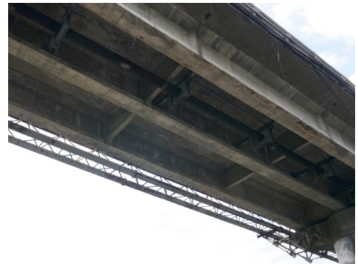
Figure 11. The surveyor can easily analyze the status of the bridge by checking the pictures taken below the deck.
