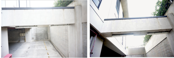
Figure 9. The side view and the bottom-up view of the frame taken by the UAV shows the possibility of implementing a UAS for bridge inspection.
