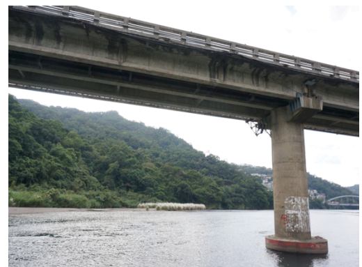
Figure 12. We also took images of the side view of the bridge so that if the beam has cracks on it the surveyor can point them out immediately.
