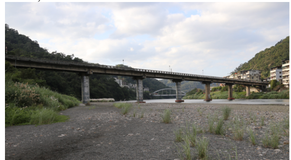
Figure 8. The Hsia-kuei Shan Bridge is a small-scale bridge, which is 8.5 m in width and 240 m in length.
