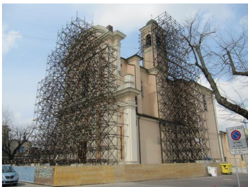
Figure 1. The church during restoration activity
