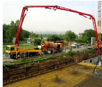
Figure 3 – Concrete Pumping in Hong Kong [25]
