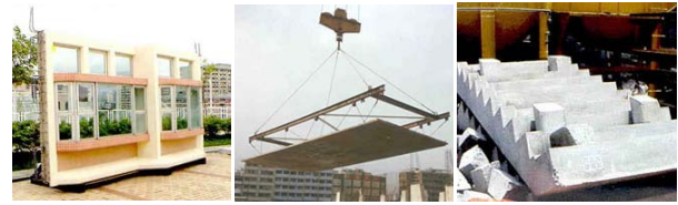
Figure 1 - Precast elements (facades, slab, and staircase) used in HA public housing [7]
