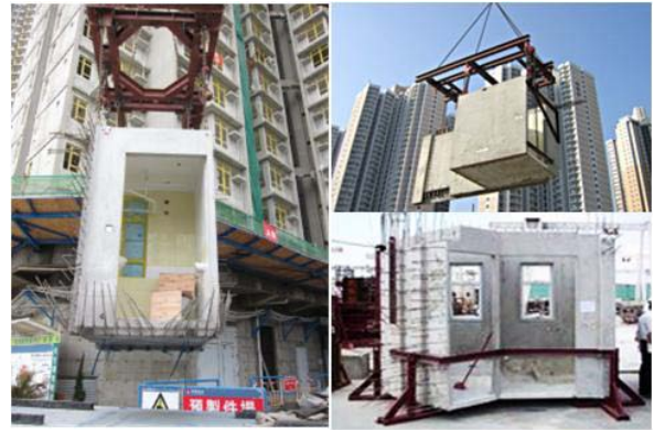
Figure 2 – Volumetric precast components (bathroom and kitchen) used in HK projects [11,12]
