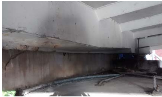
Figure 2: Photograph showing the enclosure in which the bridge bearing survey was carried out using the DiddyBorg robotic platform.
