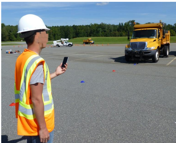
Figure 4. Ground worker with PPU.
