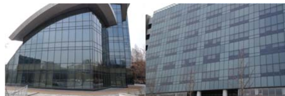
Figure 2. Curtain walls used in building façade
