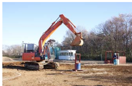
Figure 20 Remote operation on the ground
