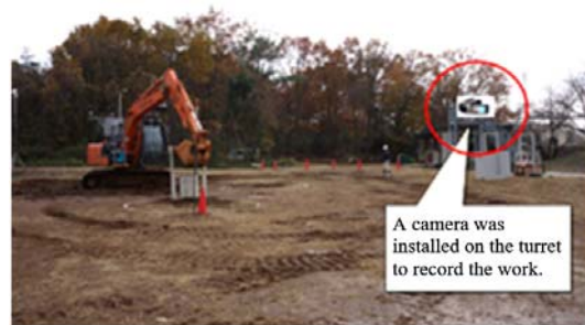
Fig. 8 Installation of work for the camera
