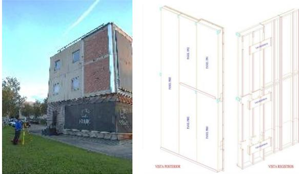
Figure 2. Left: Measuring the Kubik building strategic points. Right: Define the modules in CAD.
