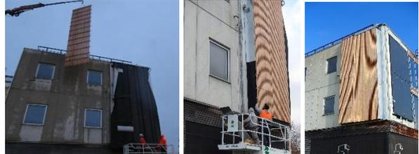
Figure 5. Left and middle: Placement and fixation of the finishing timber grid. Right: Final enclosure and perimeter finishing.
