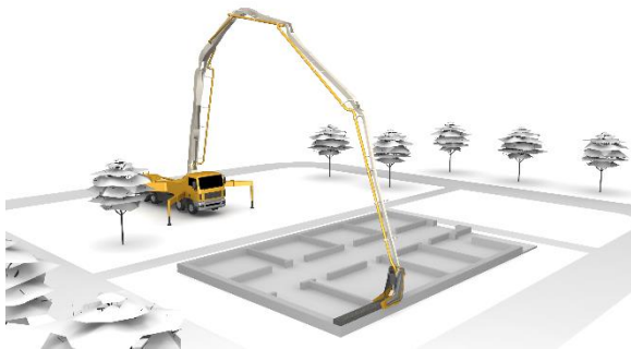
Fig. 2: Geometrically precise installation of the concrete by modified truck-mounted concrete pump
