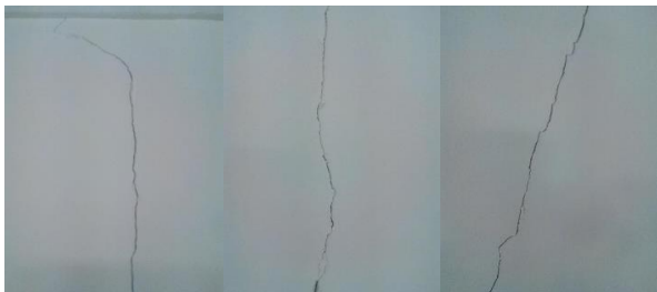
Figure 15. Sample crack images that are replaced with the acquired images
