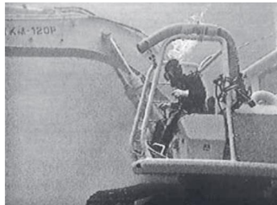
Figure 2. An excavator operated by a diver [1]
