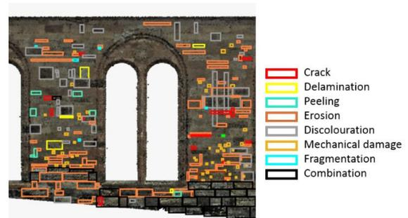
Figure 6. Defective areas labelled by surveyors
