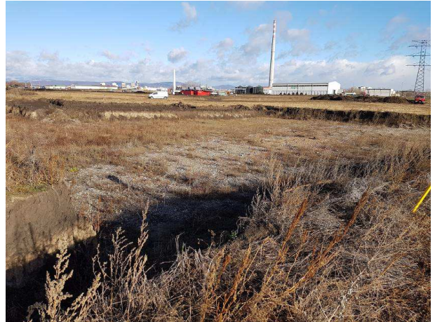
Figure 1 Preparation of excavation works, Lagoon
