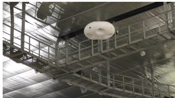
Figure 3. Inspection of Catwalk
