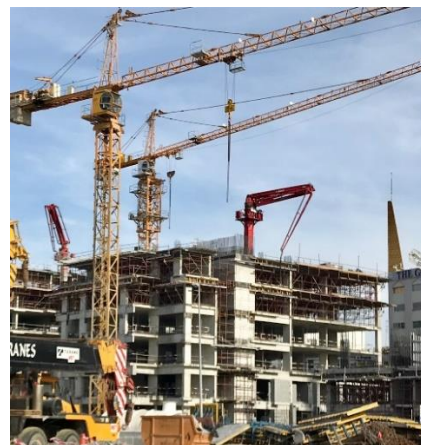
Figure 1. Tower cranes and concrete pumps used in the early stages of the construction of a high-rise building (source: the authors)
