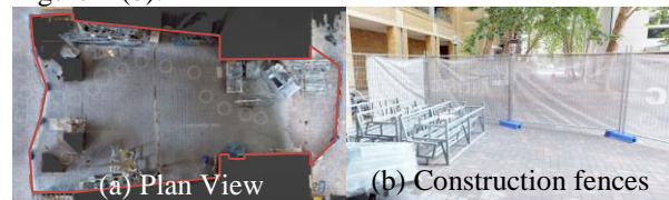
Figure 2. Quadrangle Building construction site.
