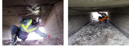
Figure 1. Status of inspection work on small bridges
