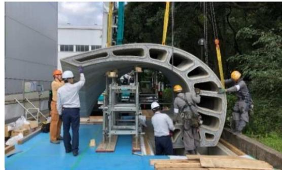
Photo 10. Erection and installation of the pieces
