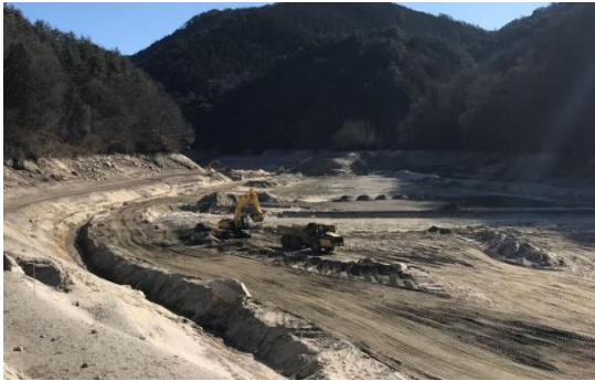
Figure 2. Construction site photo
