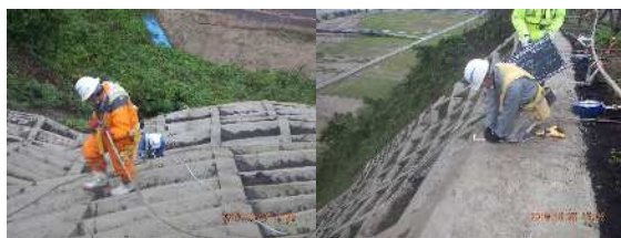
Figure 6. Status of surveying works
