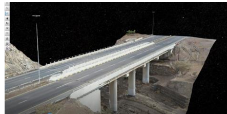
Figure 4. Bridge 3D model from LiDAR data collection
