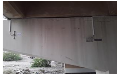
Figure 6. Mechanical remote sensors for bridge data collection
