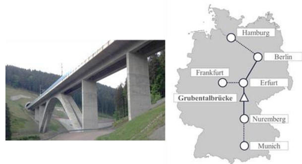
Figure 6. Railway Bridge Grubental (left) and the local placement within the high-speed rail network in Germany (right)
