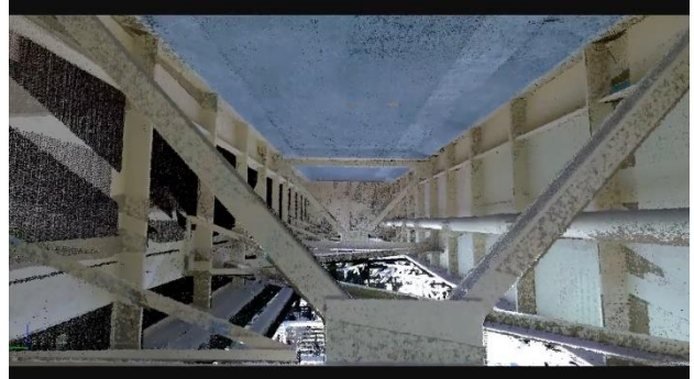
Figure 2 . Three-dimensional point groups model in bridge girder
