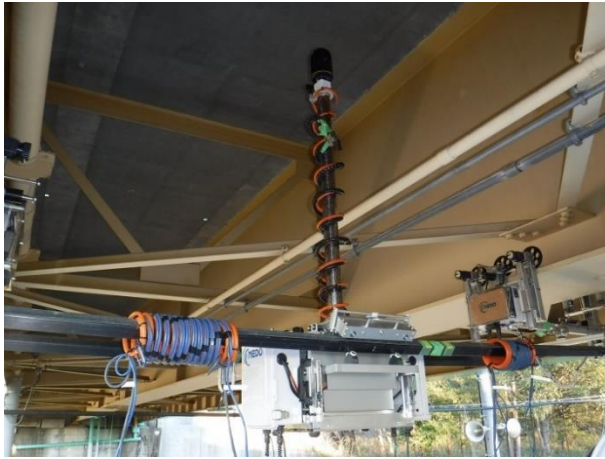
Figure 6. Turrets equipped with a three-dimensional scanner
