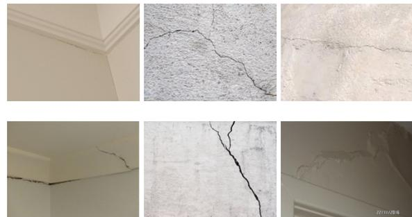
Cracks that are wider at the top or the bottom may indicate that there has been foundation movement, with the direction of the widening indicating the likely direction of the movement.
