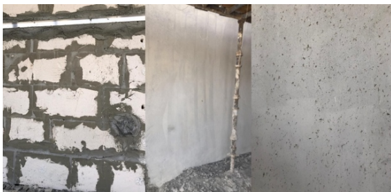
Figure 3. 3 stages of construction
