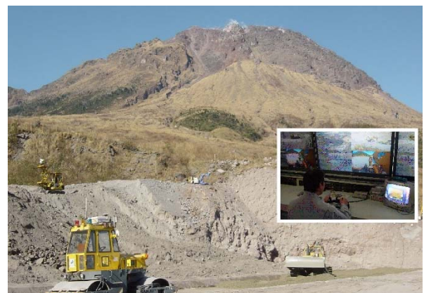
Figure 1. Status of unmanned construction
