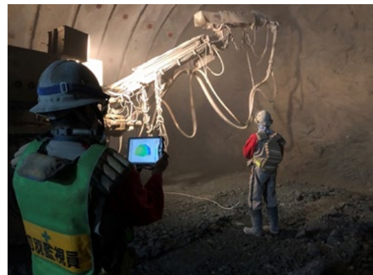
Figure 6. Face monitoring personnel monitors the face
